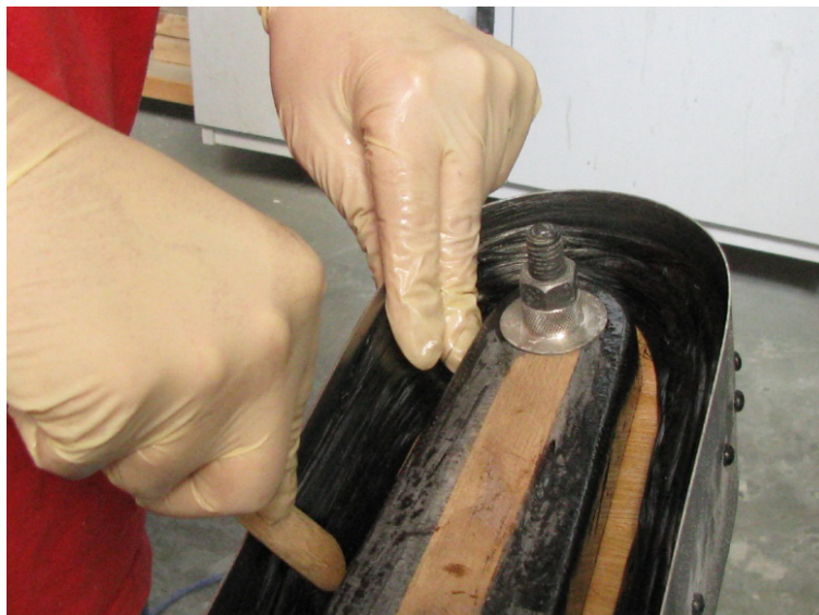
Fig 8: Carbon Rope Lay-up in Progress
