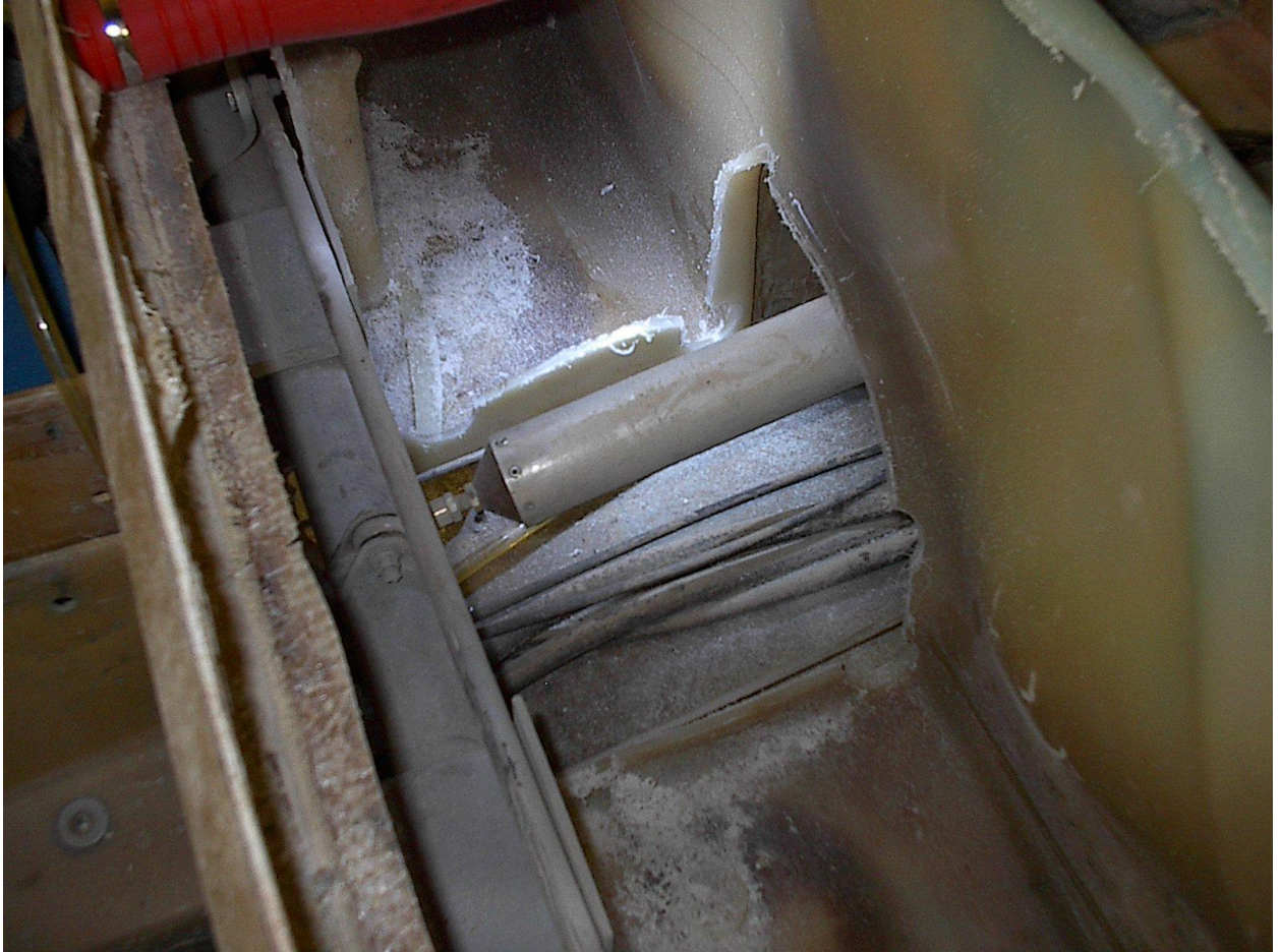
Figure 6 Carefully cutting around the controls.
