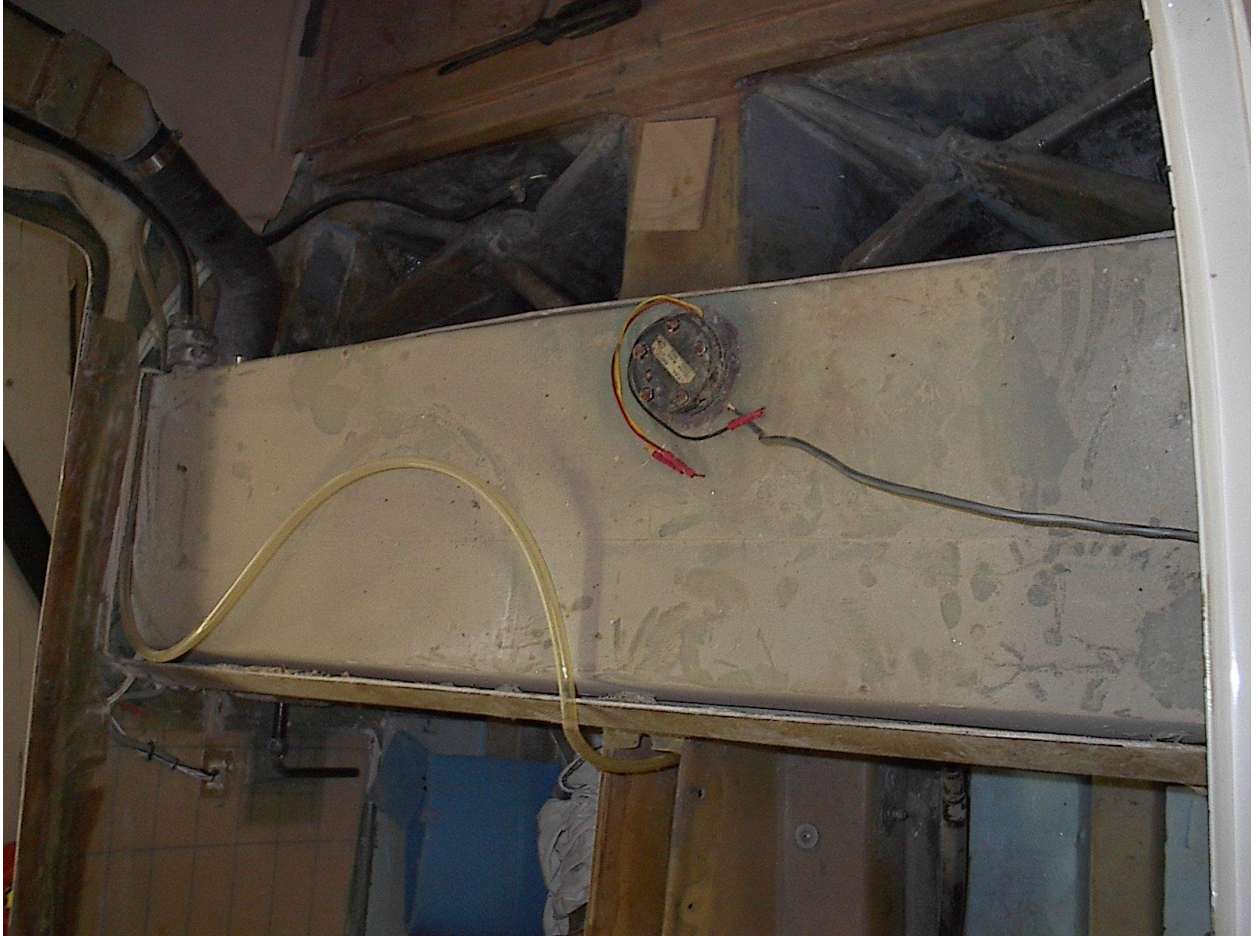
Figure 4 Tank top now exposed
