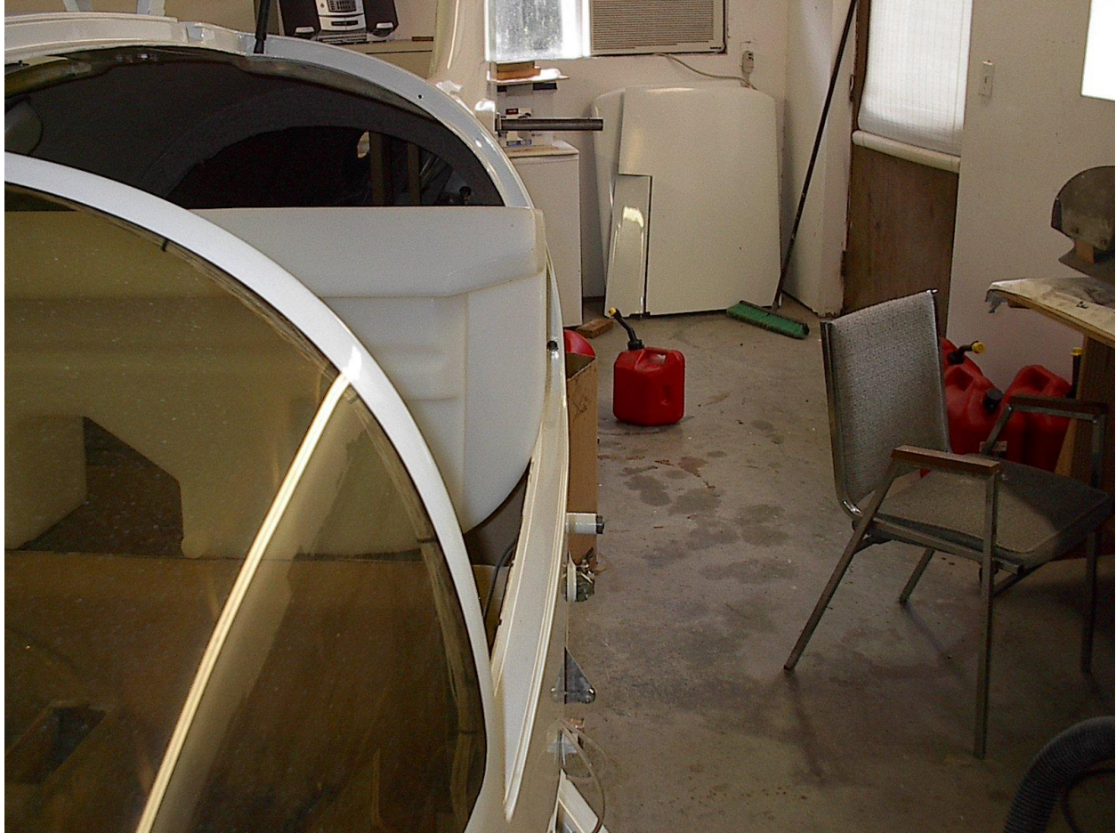
Figure 7 The side rails need to be cut out for the new tank just a bit. I recommend cutting out about half the flange.
