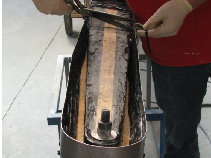
Fig 7: Carbon Rope Lay-up Showing Tapered Void to be Filled
