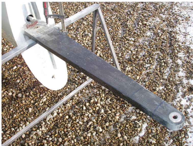
Inspect spar tang on all four surfaces
